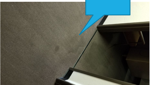
WORN CARPET OVER UNEVEN SURFACES THROUGHOUT THE FACILITY
