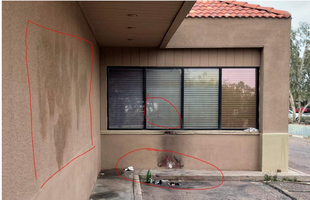
Figure 8 - Fire damage, Trash, Broken glass, Graffiti on the back side
