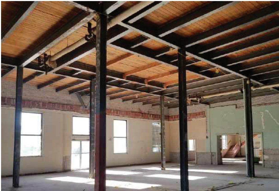
Federal Building Renovation
