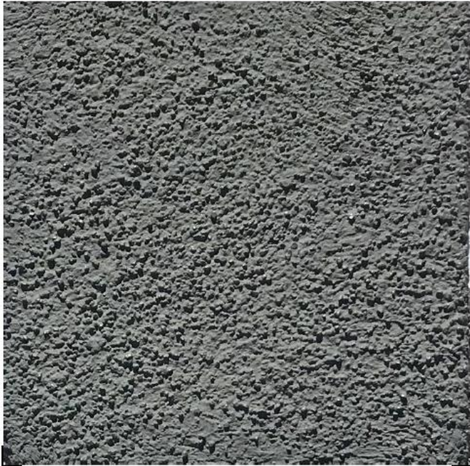
1.1 STC1: STUCCO, SAND FINISH TEXTURE WITH REVEALS AS SHOWN ON ELEVATIONS (UNCOLORED)
