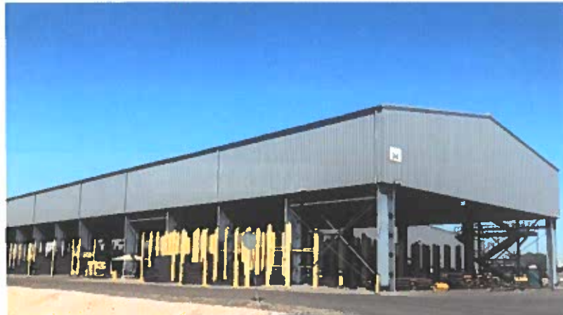
AZ1 – Rebar Finished Goods (Typical style to match on AZ2)
