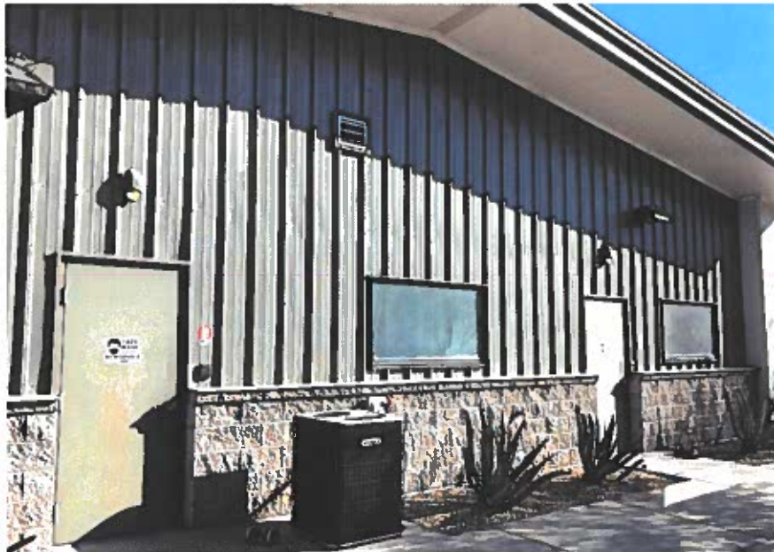
AZ1 – Office Building (Typical style to match on AZ2)
