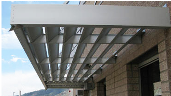
12" deep aluminum frame canopy system; attached to building walls, see exterior elevations for locations
