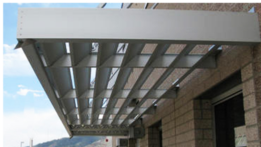
12" deep aluminum frame canopy system; attached to building walls, see exterior elevations for locations
