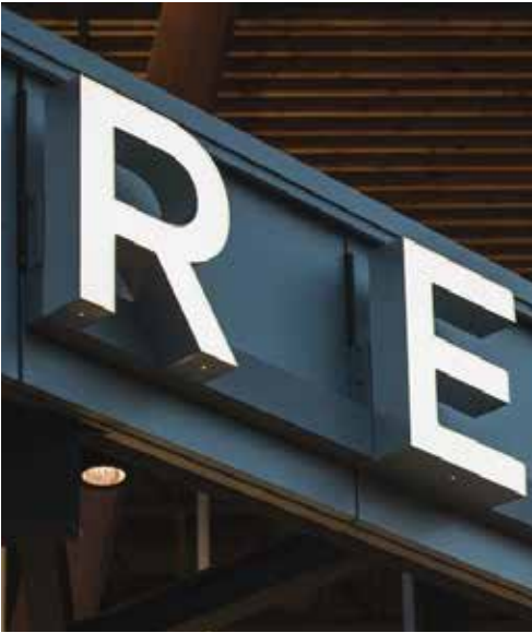
Pan Channel Letter Internally Illuminated
