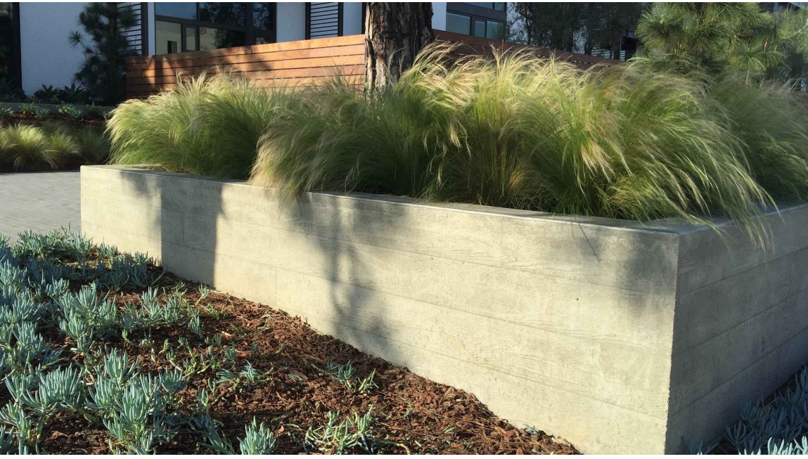
Board Formed Concrete Terrace Walls
