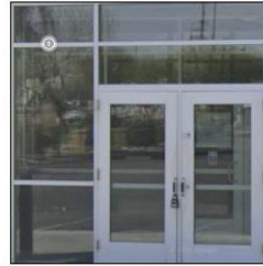
EXISTING MULLIONS KAWNEER ALUMINUM CLEAR ANODIZED
