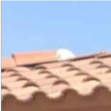
EXISTING CLAY ROOF TILE PATCH AND REPAIR AS NEEDED
