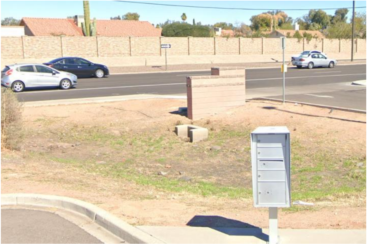
1. Northeast screen wall
