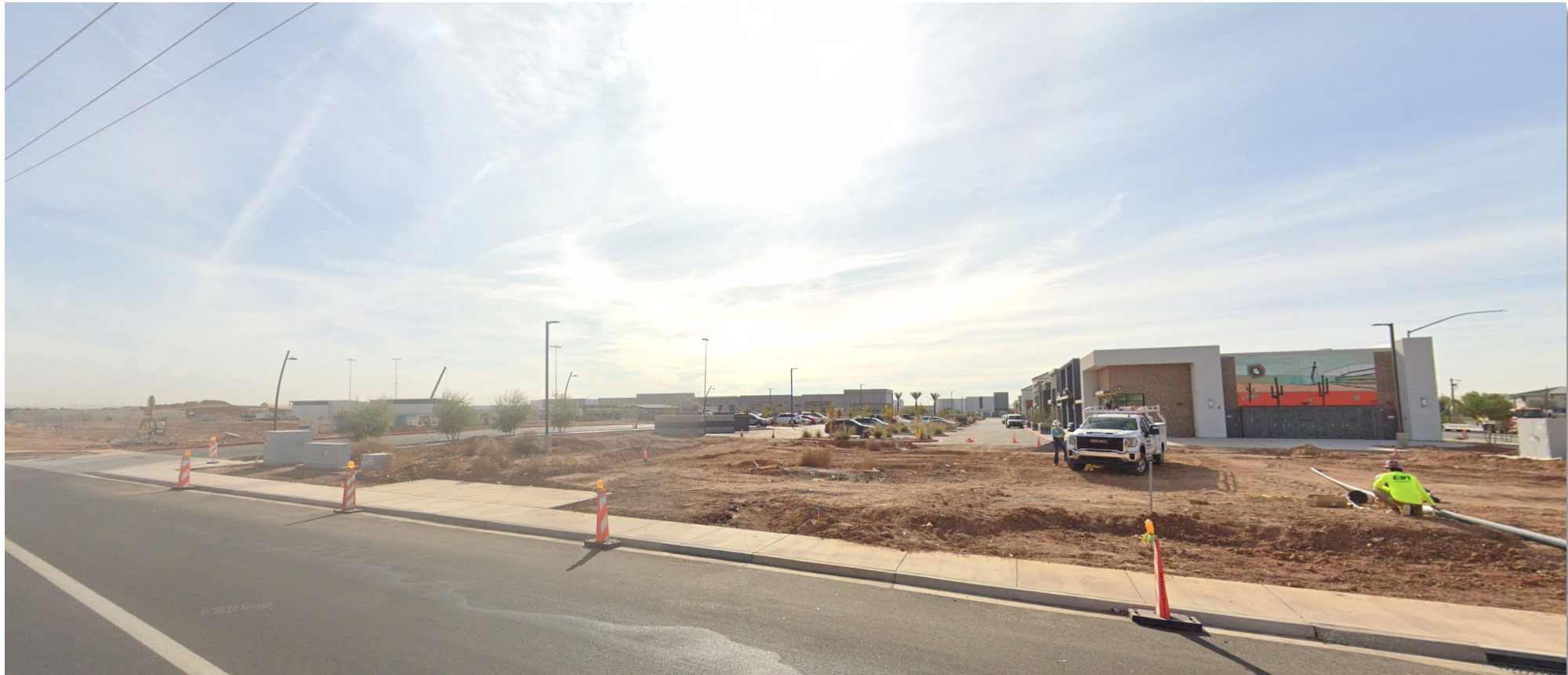
Looking south toward the site from Warner Road
