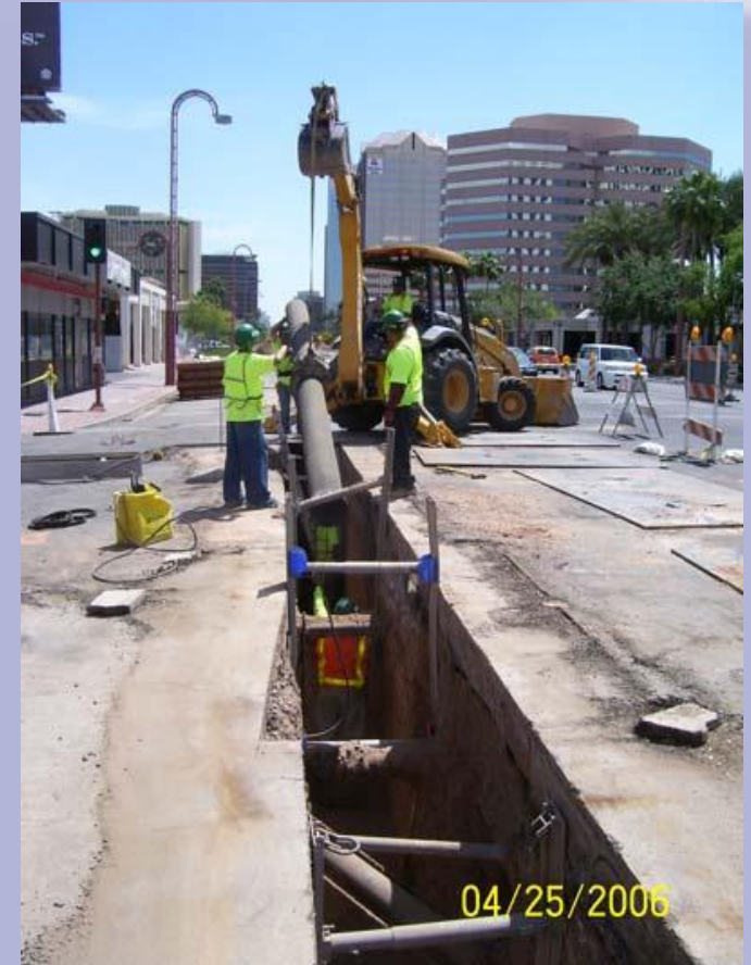
Sewer line relocation
