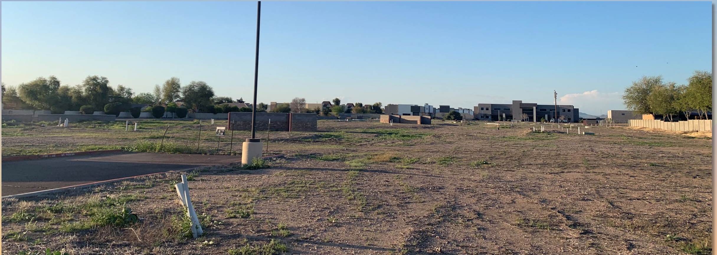
Looking northwest from mid-point of Project Site at east side
