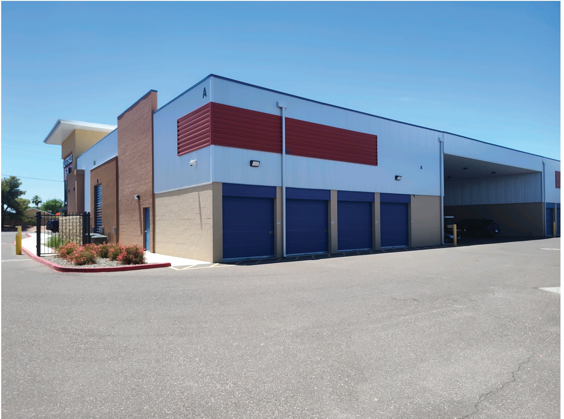
EXISTING BUILDING INTERNAL YARD VIEW
