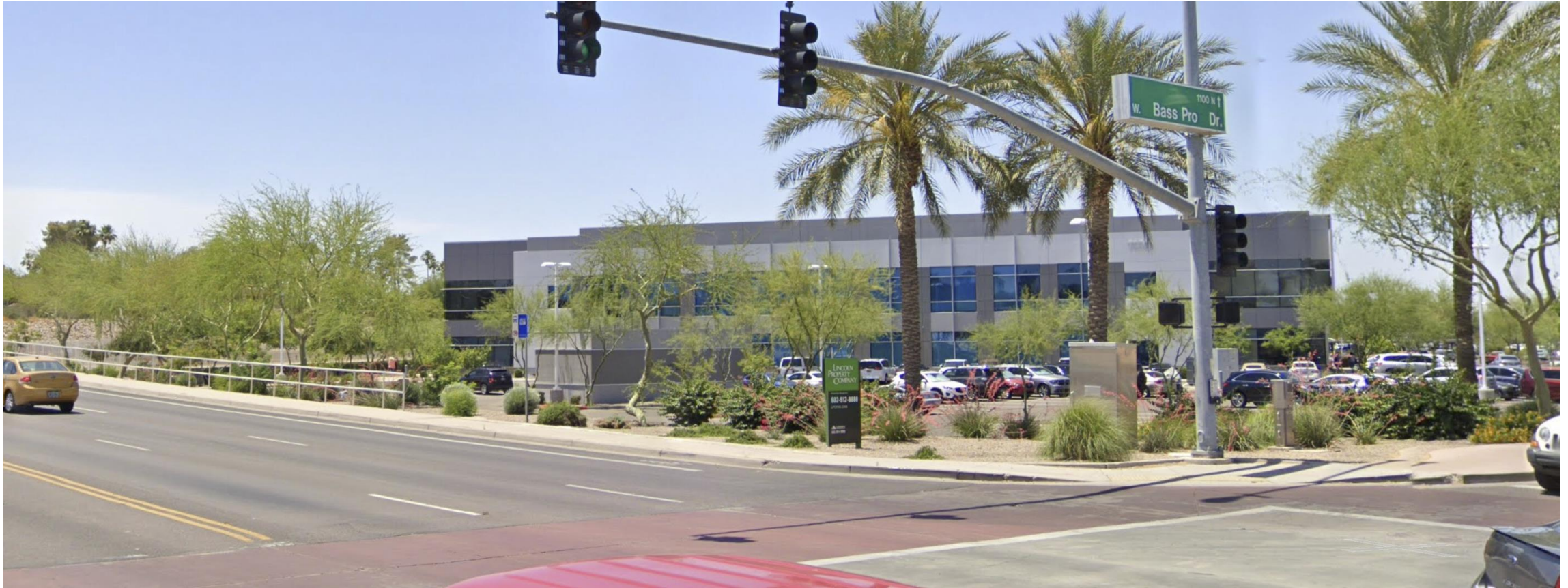
Looking southwest from Alma School Road & Bass Pro Drive
