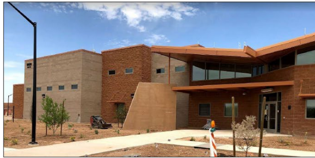
Existing Operations Building
