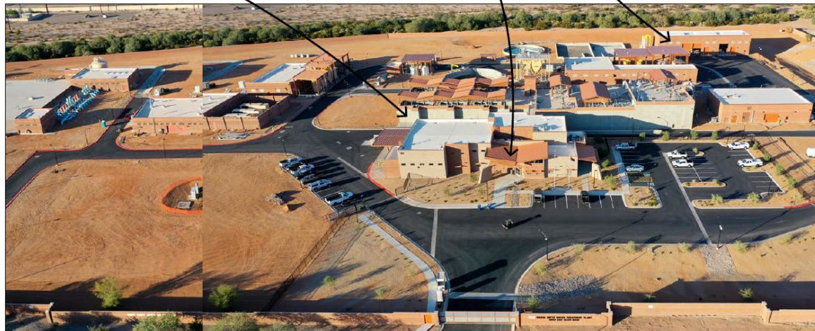
South Aerial View
