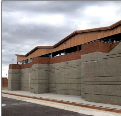
Existing Filter Complex
