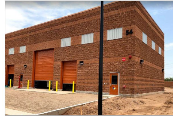
Existing Dewatering Building (typical façade treatment for all process buildings)
