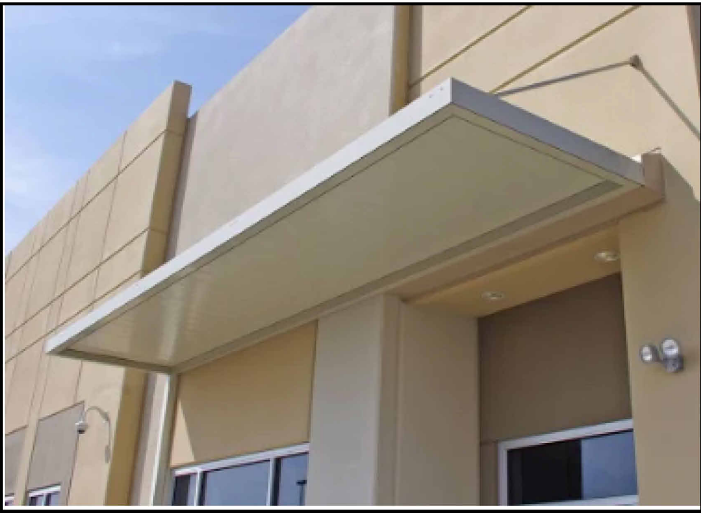
PREFINISHED METAL AWNING (CN-1)
