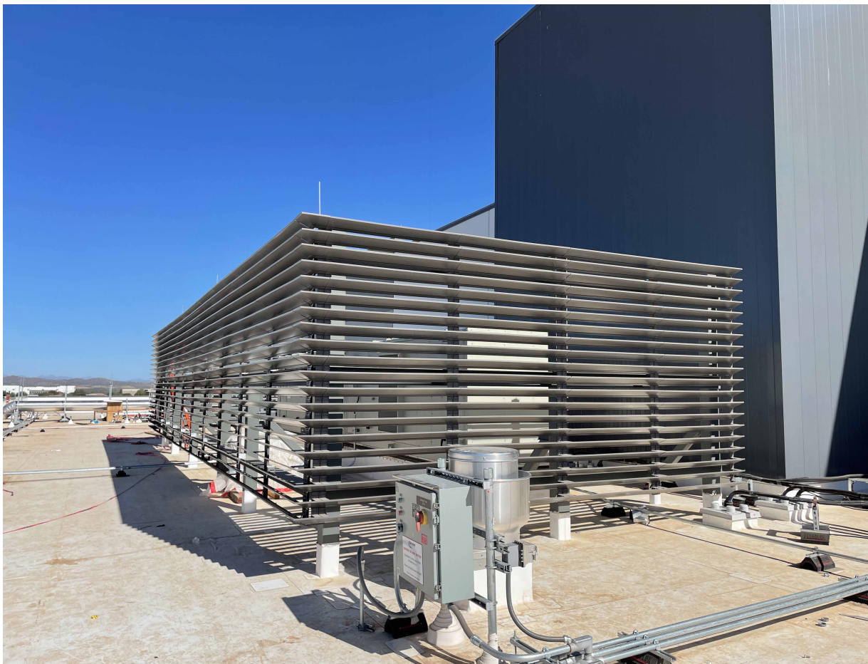
LOUVERED EQUIPMENT SCREEN
