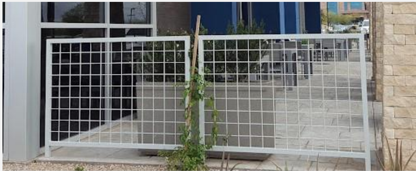
PATIO RAILING & WIRE MESH
