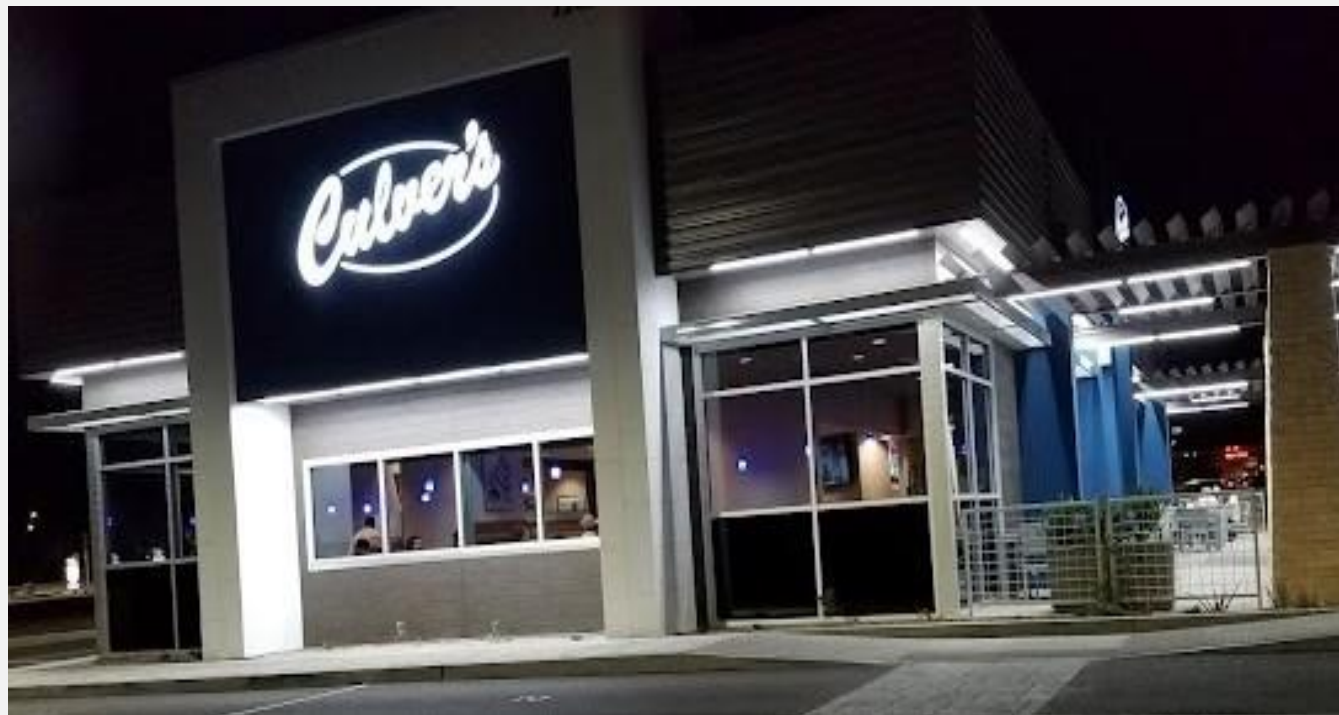
EXTERIOR LIGHTING LINEAR LIGHT FIXTURES
