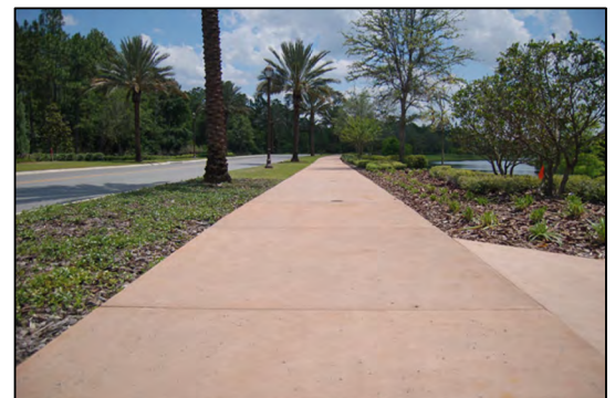
Colored Concrete Crosswalks
