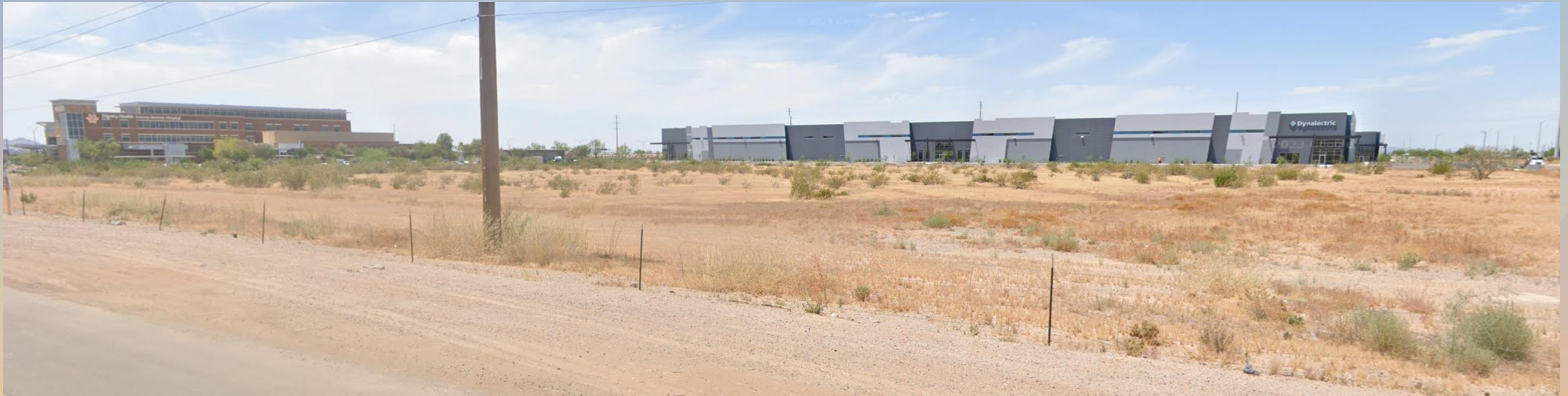
Looking southwest from Ellsworth Road
