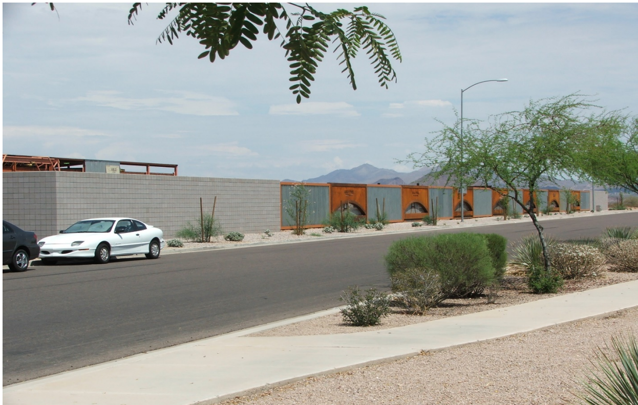
Figure 3 – West Side of Norwalk After (South View)
