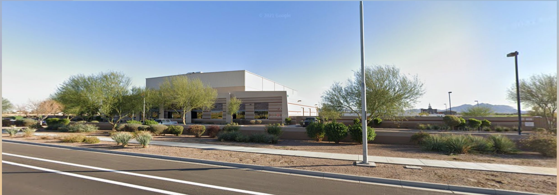
Looking southeast at the existing Metso site
