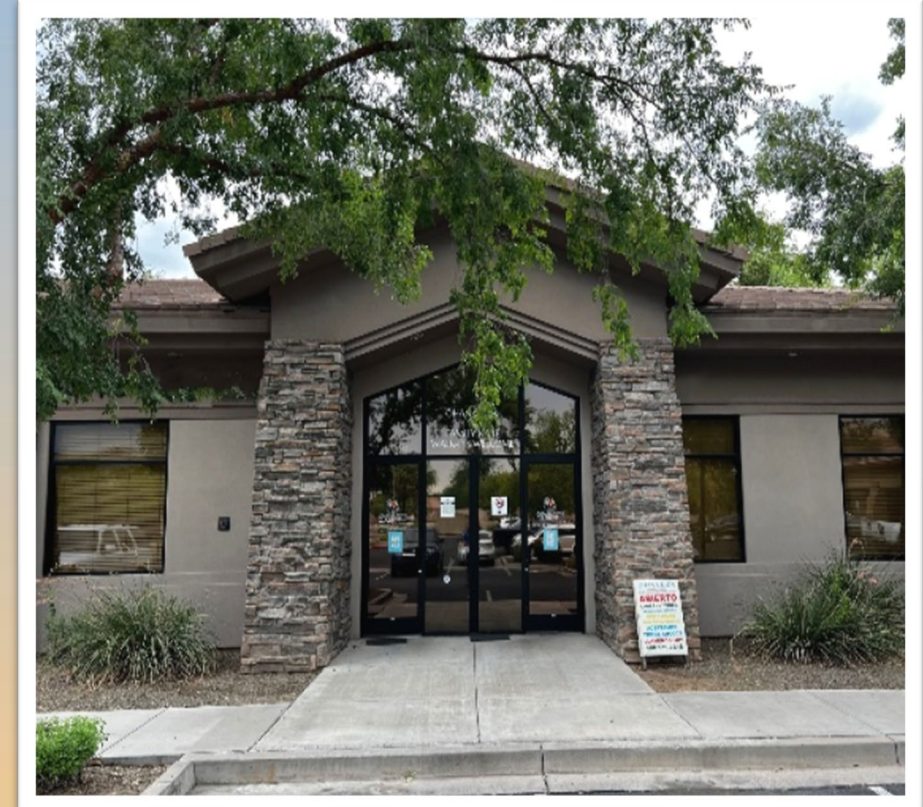
Looking towards the Suite 103: All previous signage has been removed
