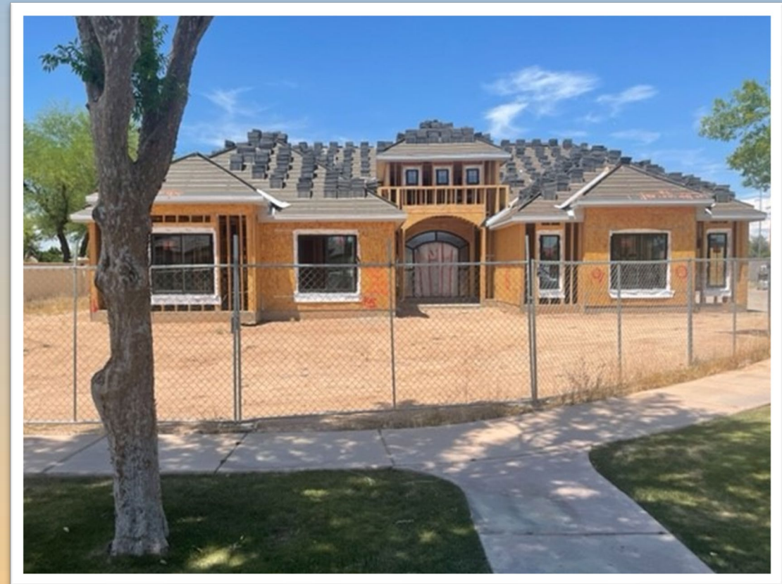
Looking north towards the residence
