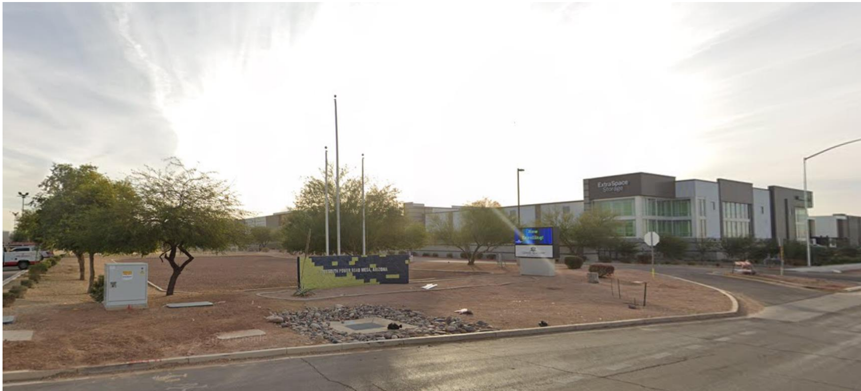
Looking East from Power Road
