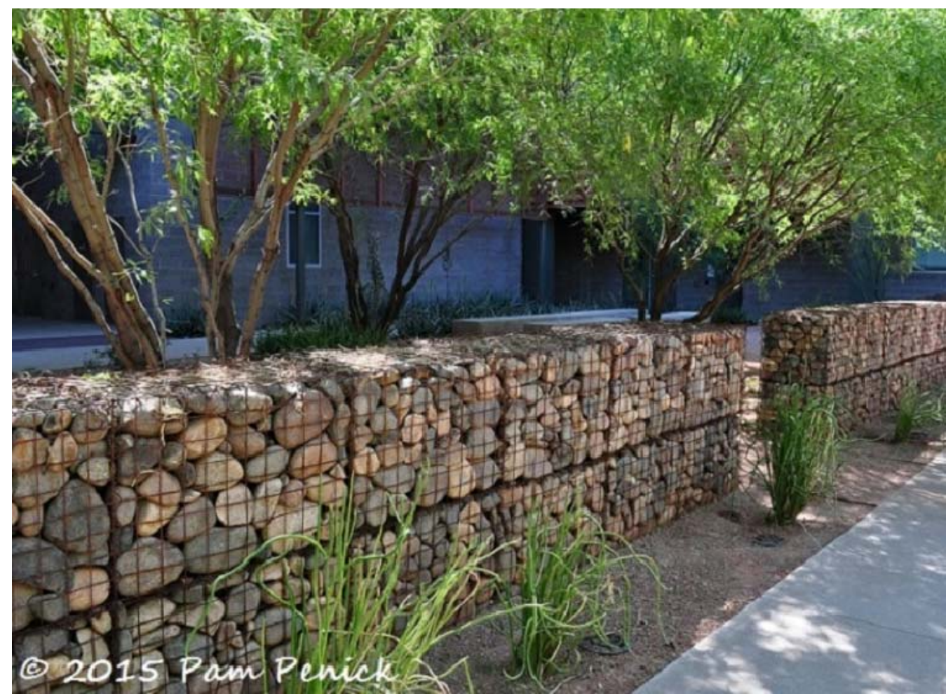
STONE FILLED GABION BASKET ENTRY FEATURE
