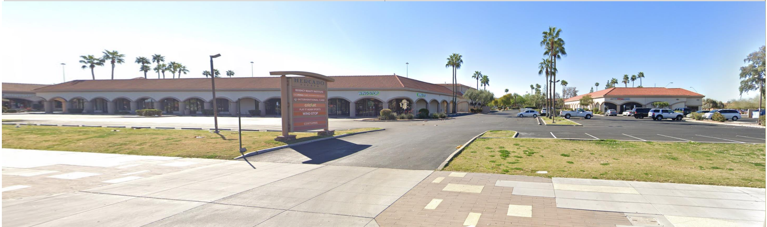
Looking south towards the site
