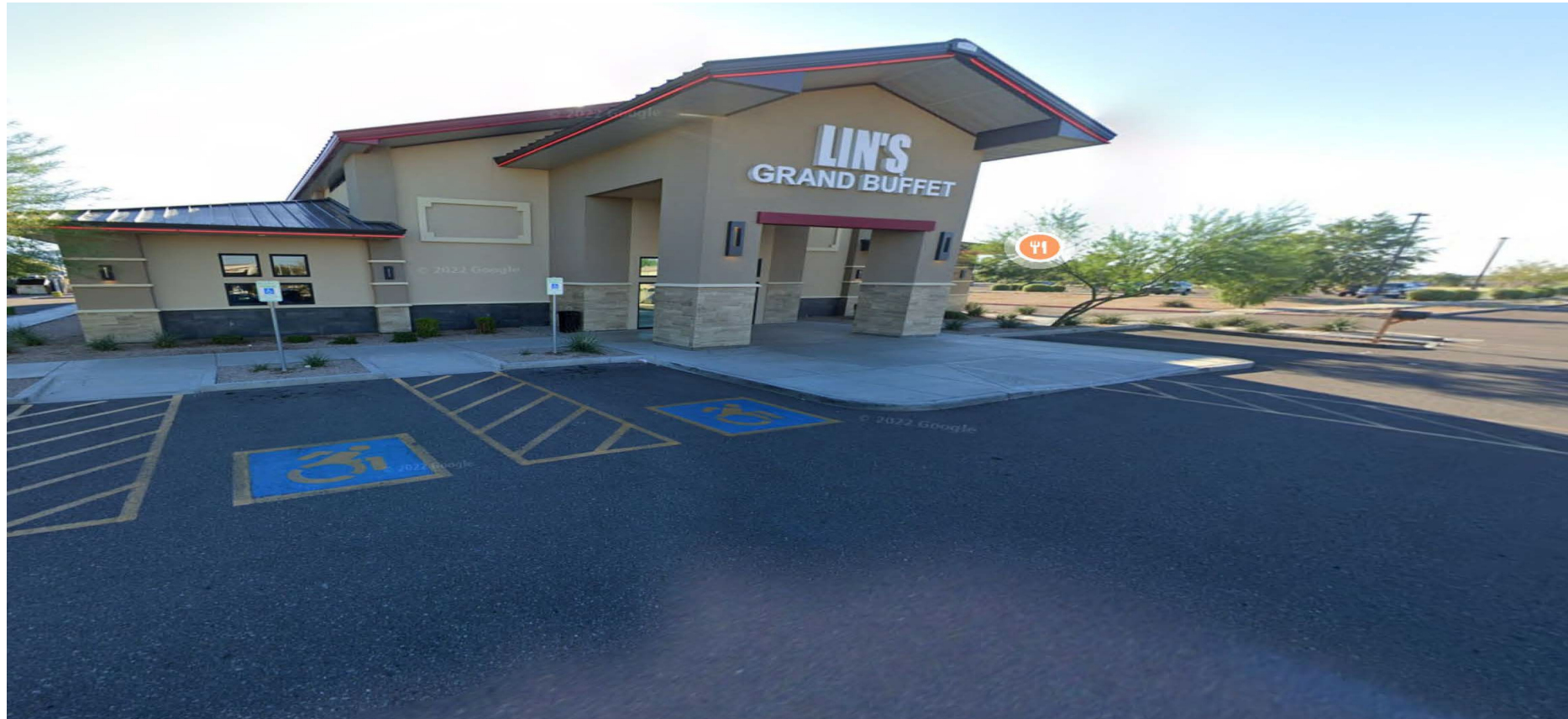
3) EXISTING LINS RESTAURANT
