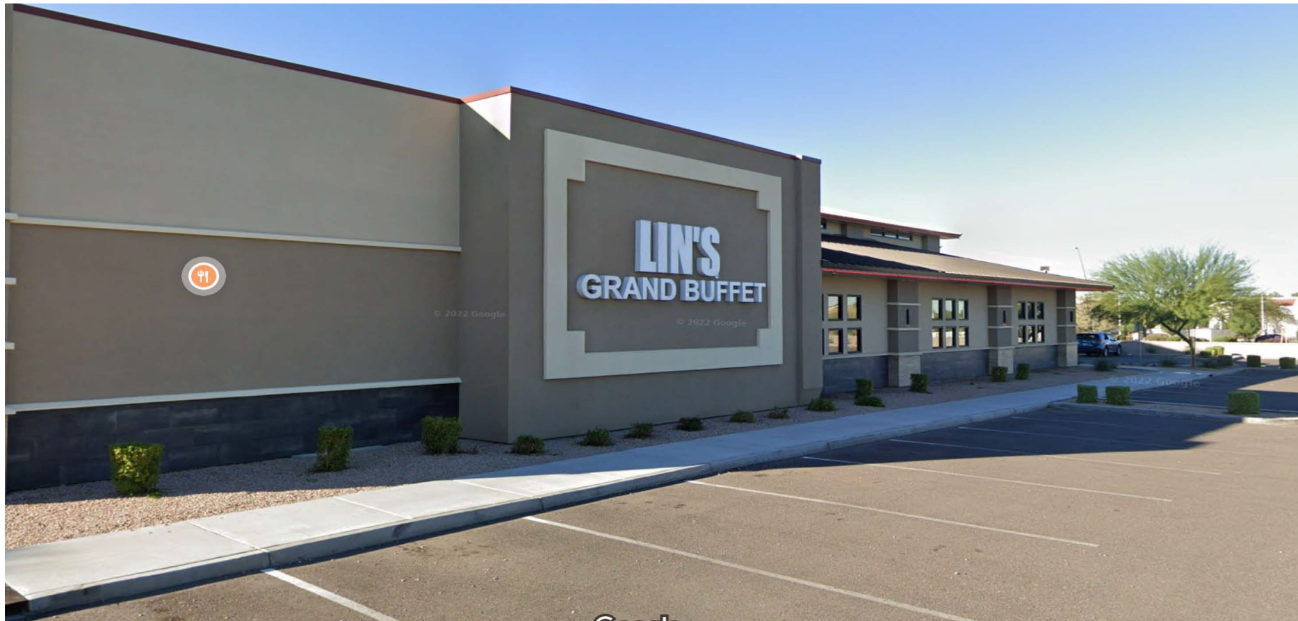
4) EXISTING LINS RESTAURANT
