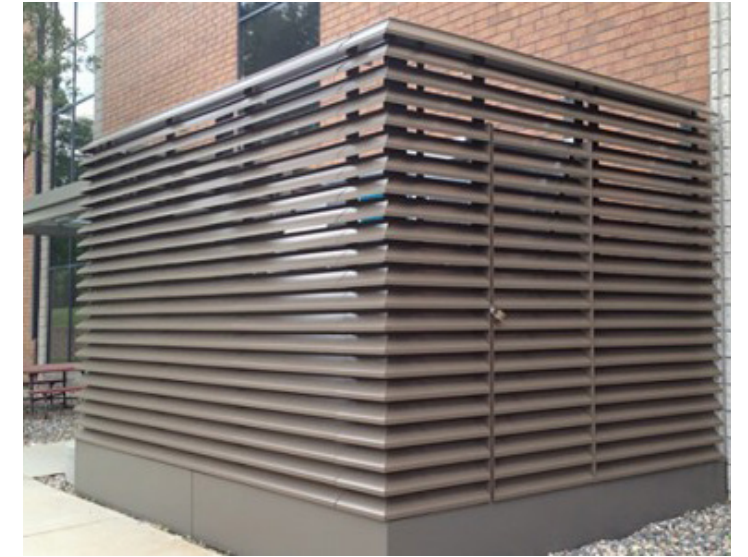
Ground Mechanical Screen
