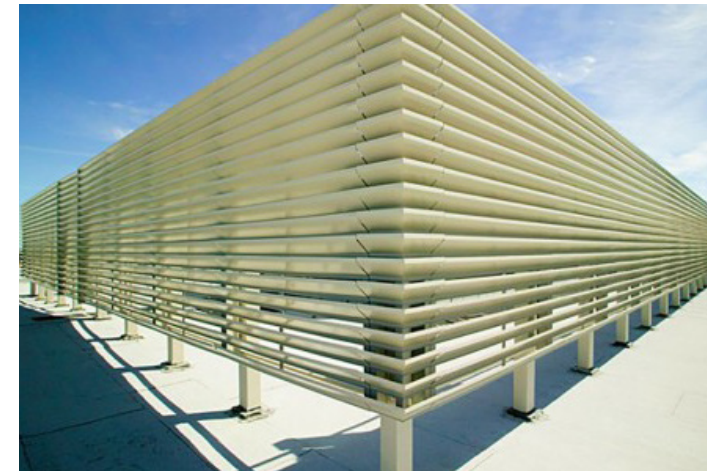
Rooftop Mechanical Screen
