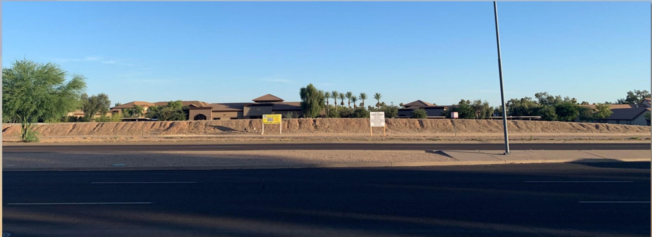
Looking south from Main Street
