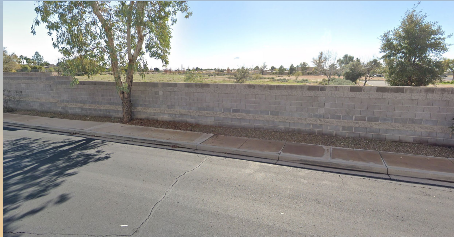
Looking southeast from Encanto Street
