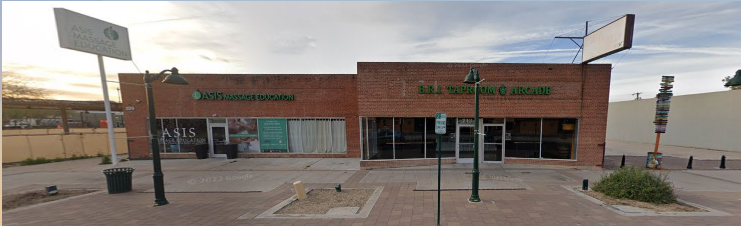
Looking south towards the site from Main Street
