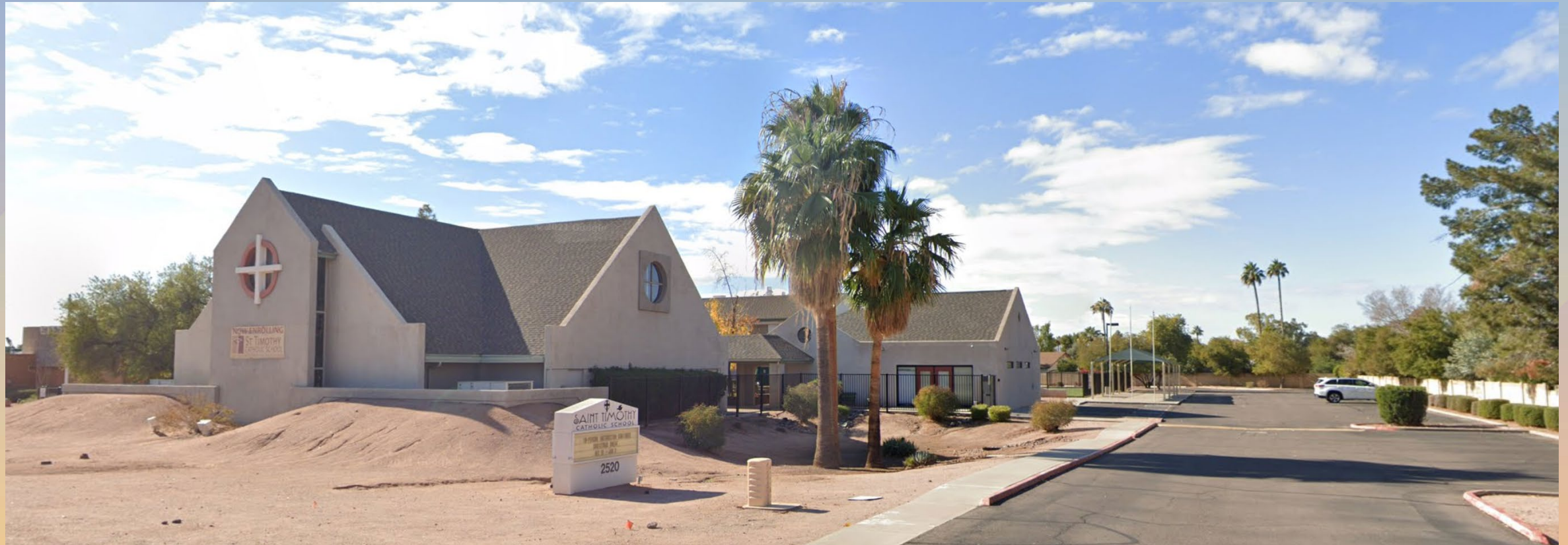
Looking southwest from Alma School Road
