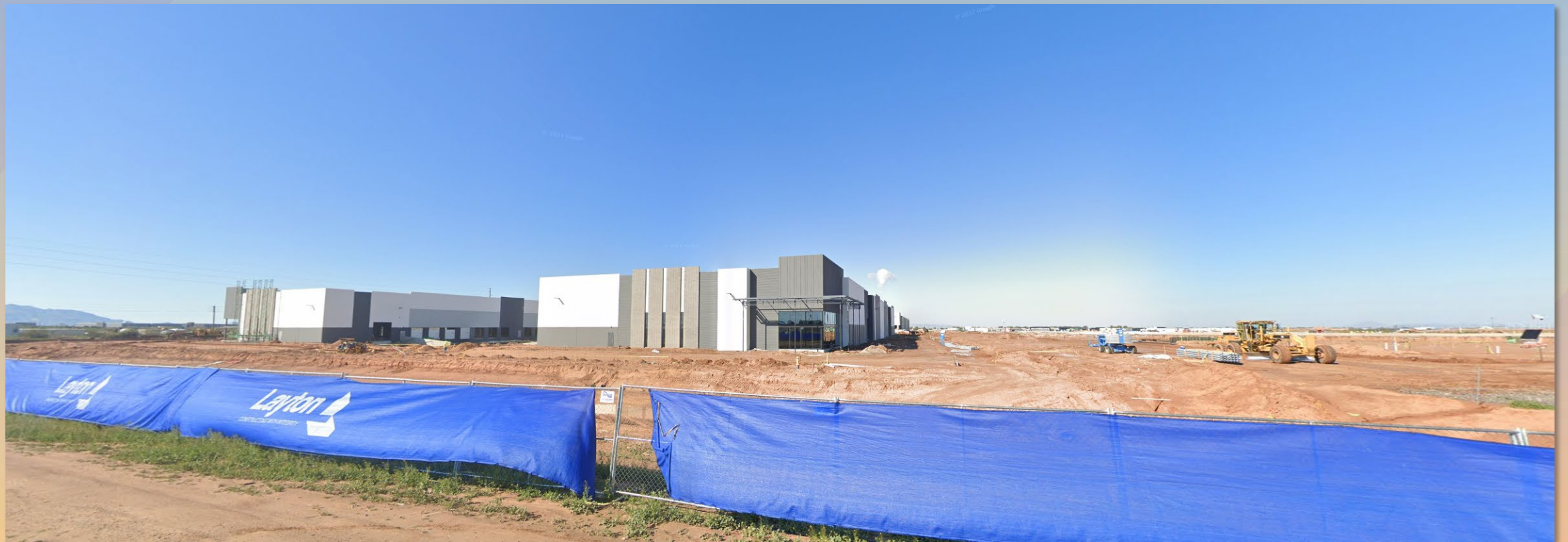
Looking southwest from S Sossaman Road
