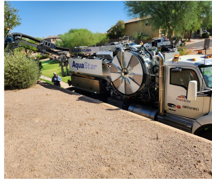
Sewer Line Inspection and Cleaning Program
