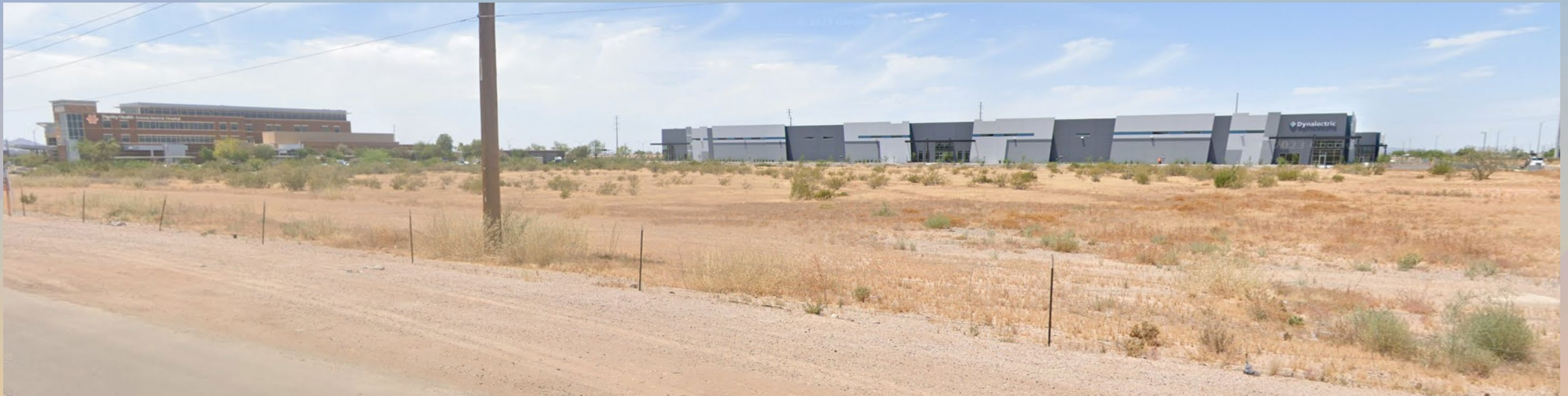
Looking southwest from Ellsworth Road
