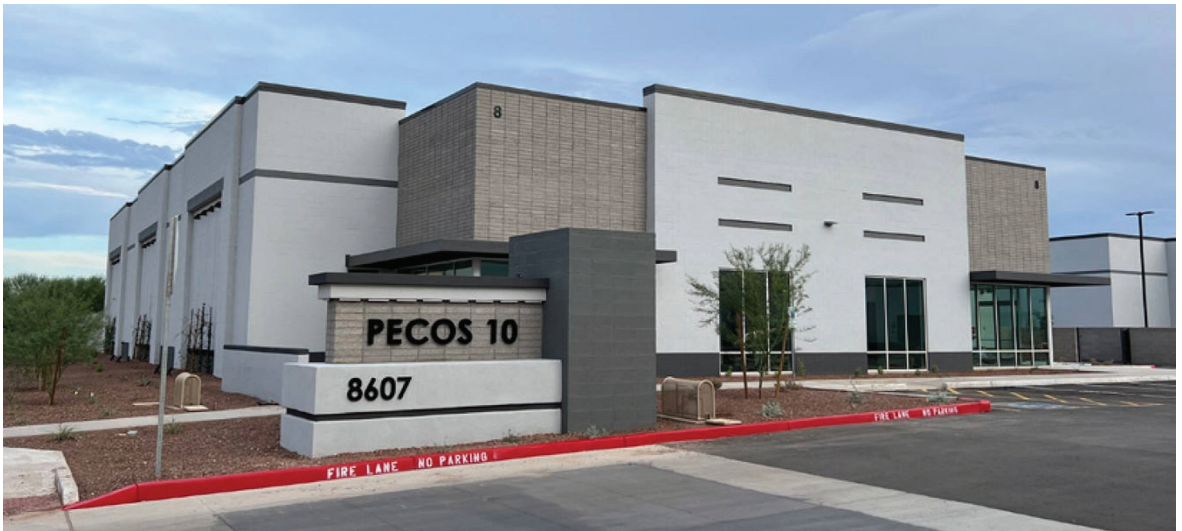
Image 2: Pecos 10 Industrial Condos (APN# 304-62-970) Existing office/warehouse condominium property located west of the proposed development, utilizing similar materials of concrete masonry and stucco, as well as similar color palette.
