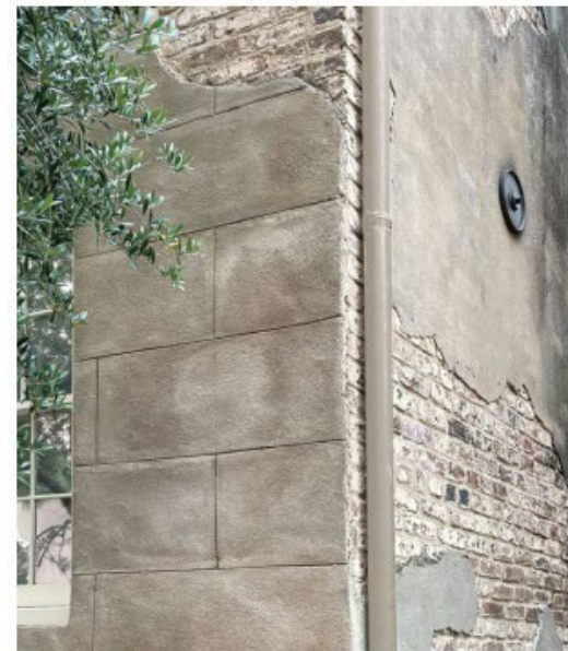
Figure 2c. Stucco has been used to imitate a number of building materials for many centuries. Seen here, stucco was applied to a brick structure and scored to represent a stone façade. Photo: John Sandor, NPS.
