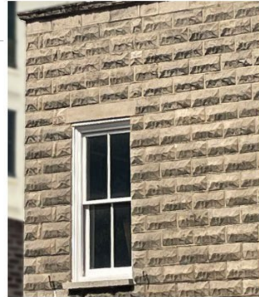
Figure 2a. Casting concrete blocks to mimic quarried stone was a popular late 19th- to mid 20th-century technique. Concrete masonry units could be completed by local craftsmen, saving time and shipping costs. Photo: John Sandor, NPS.
