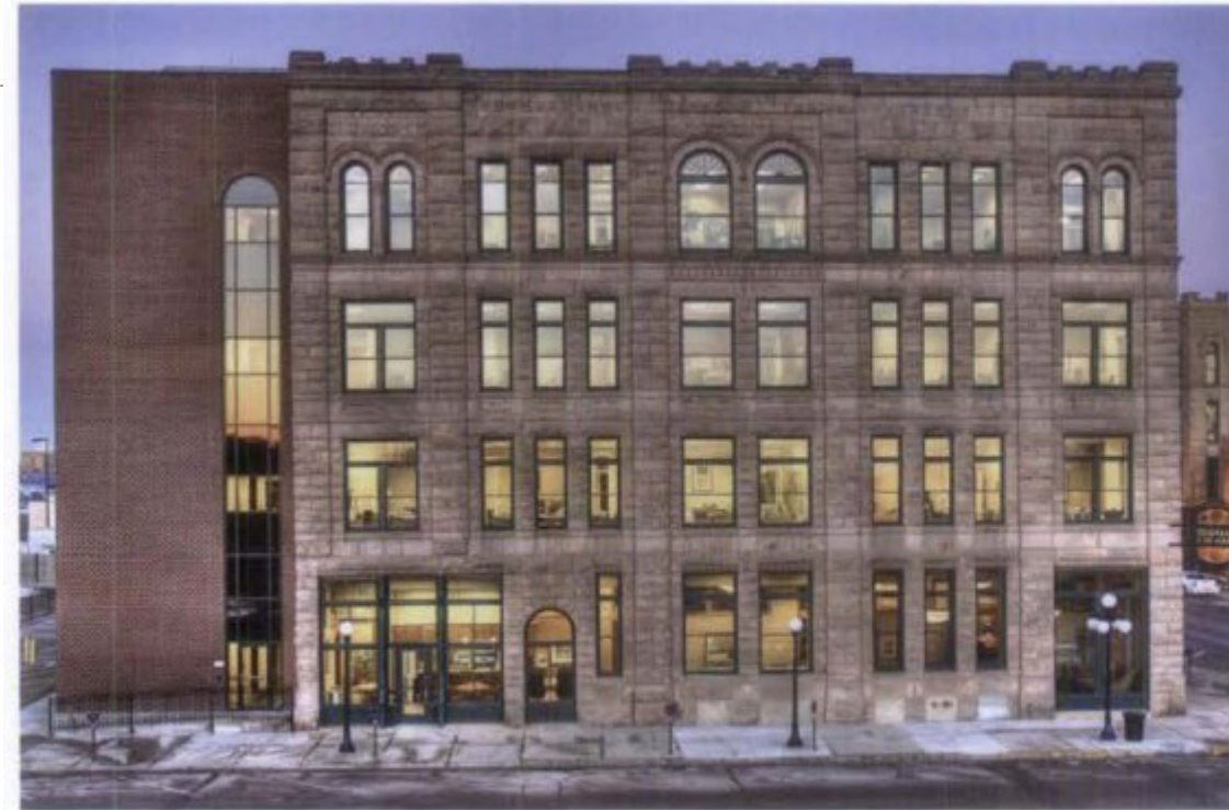
Figure 27. Although the new brick stair/elevator tower (left) is not visible from the front (right), it is on a prominent side elevation of this 1890 stone bank. The compatible addition is set back and does not compete with the historic building. Photos: Chadd Gossmann, Aurora Photography, LLC.
