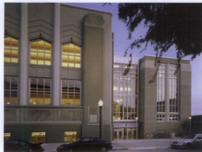
Figure 1. The addition to the right with its connecting hyphen is compatible with the Collegiate Gothic-style library. The addition is set back from the front of the library and uses the same materials and a simplified design that references, but does not copy, the historic building. Photo: David Wakely Photography.
