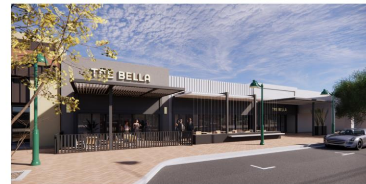
MT-03 DESCRIPTION: SHEET METAL FLASHING, METAL ACCENTS, FENCE, GATES, PLANTERS PRODUCT: B.O.D. PAC CLAD PERFORMANCE COATING FINISH/ COLOR: MATCH ADJACENT OR DARK BRONZE 614354
