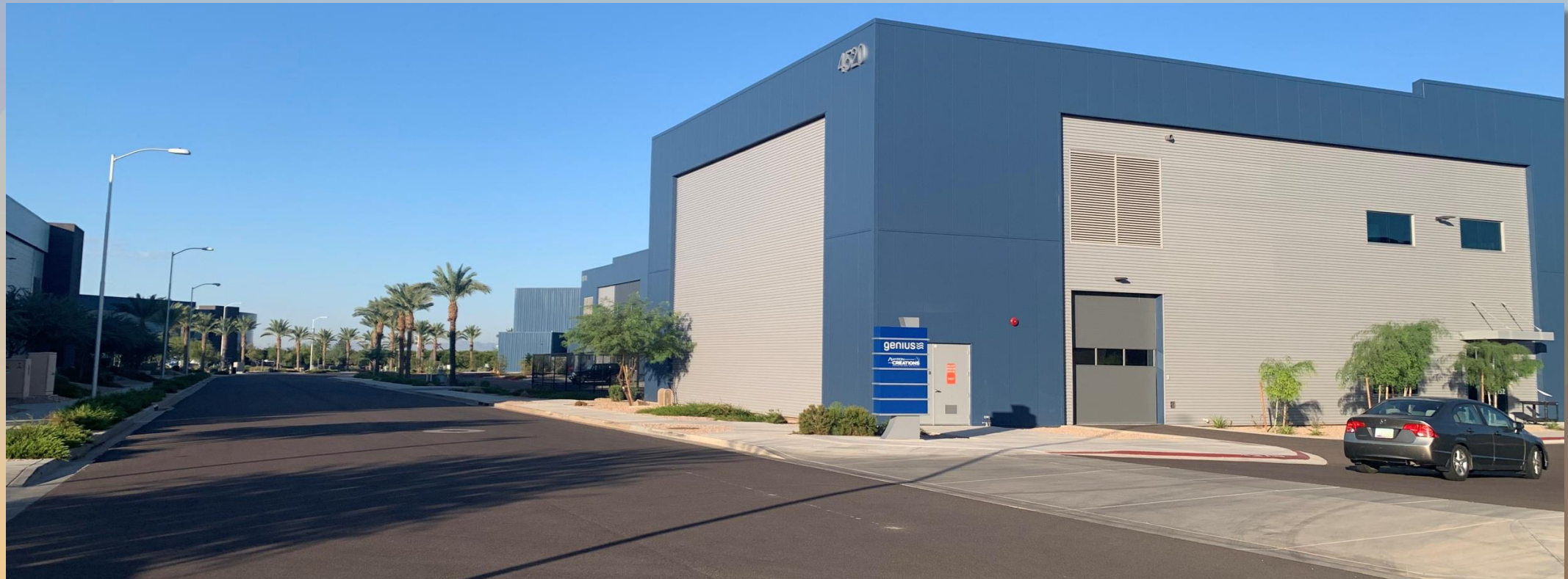
Looking west at the north side of Mallory
