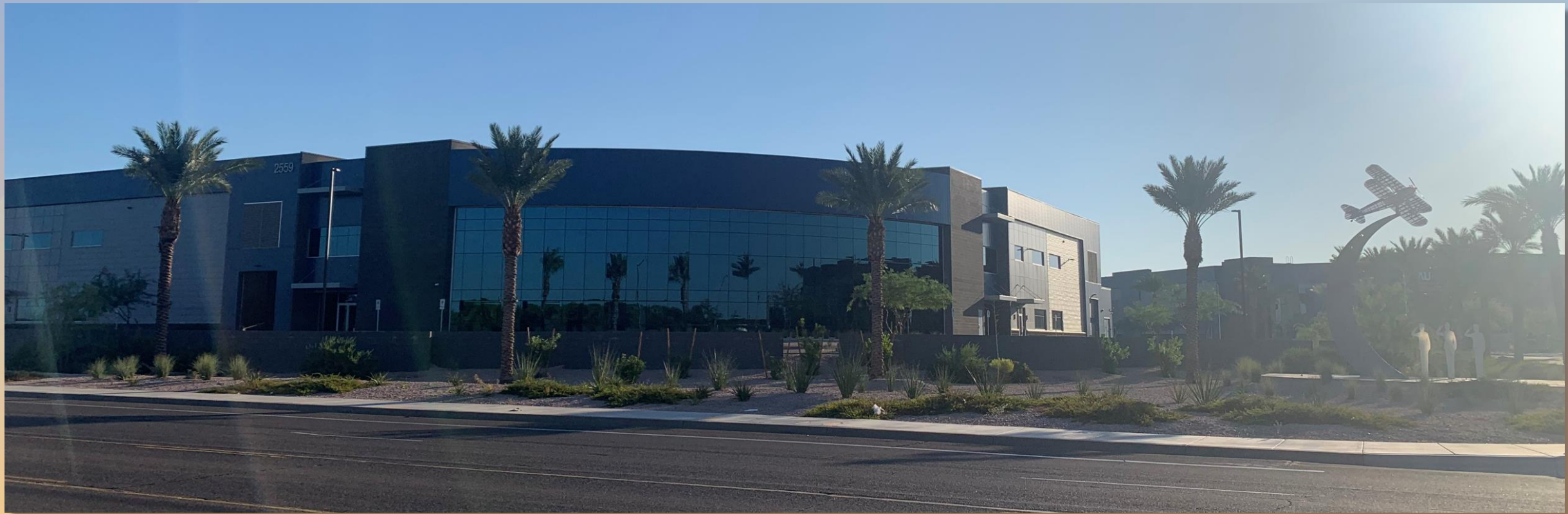
Looking east at the northeast corner of Greenfield Road and Mallory
