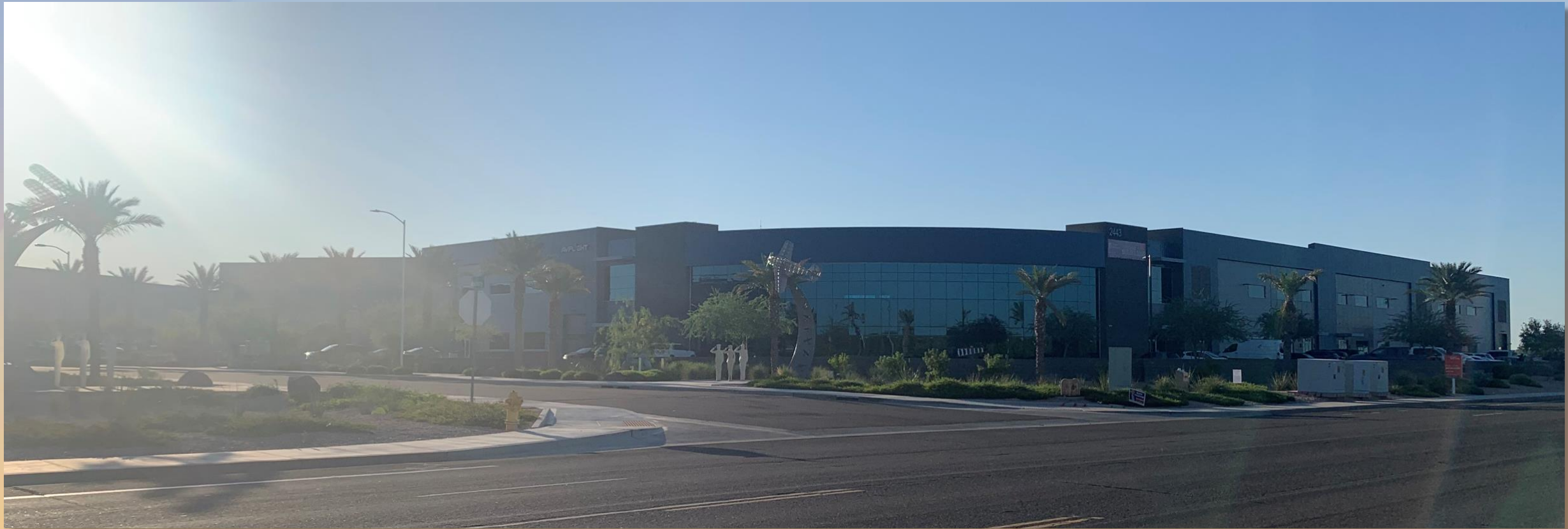
Looking east at the southeast corner of Greenfield Road and Mallory
