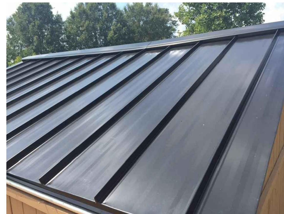
5 Standing Seam Roof SCALE: NTS
