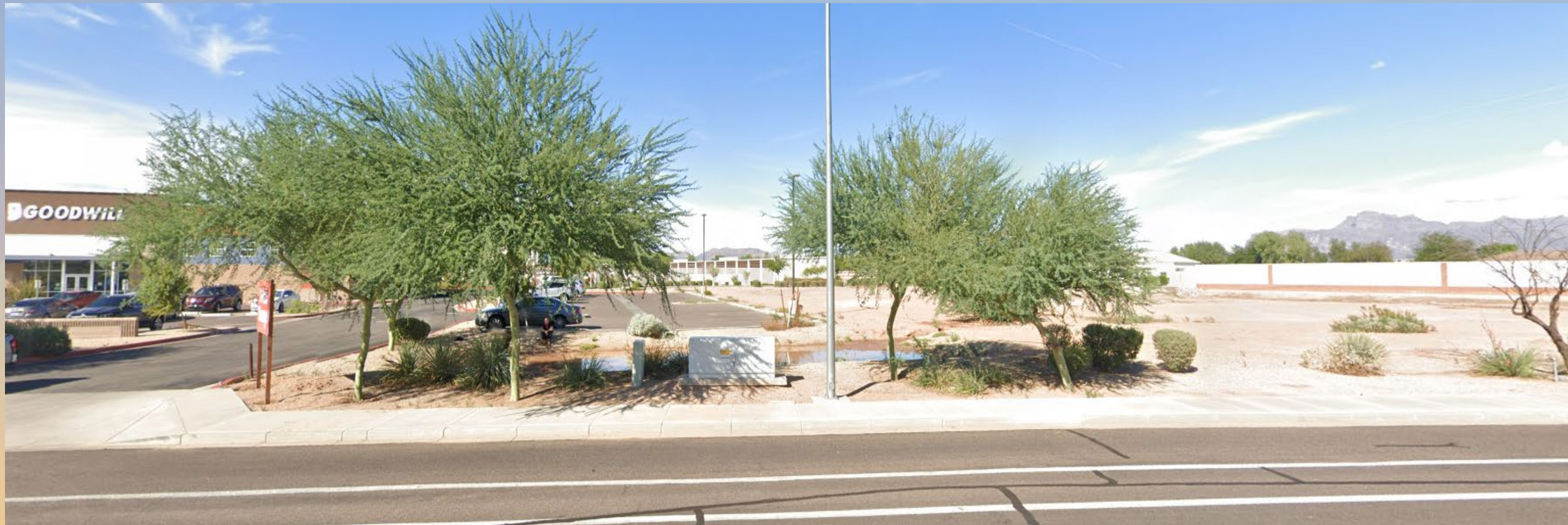
Looking northwest from Guadalupe Road
