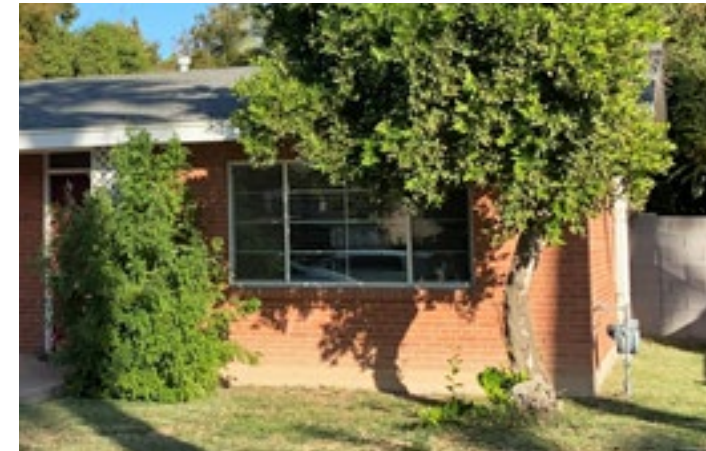
541 N. Grand (The foundation wall shown here uses different materials to visually distinguish it from the main wall)
