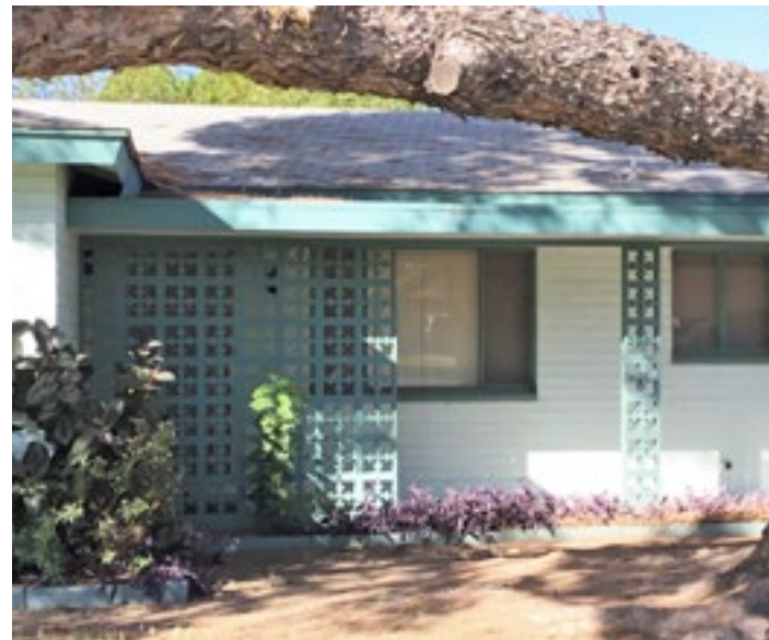
234 N. Fraser Dr. (The breezeblock elements on this porch contribute to the character of the house)
