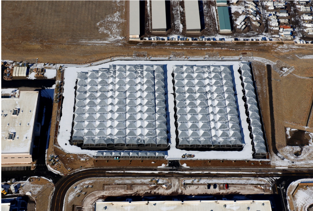
AutoNation Stack Lot
