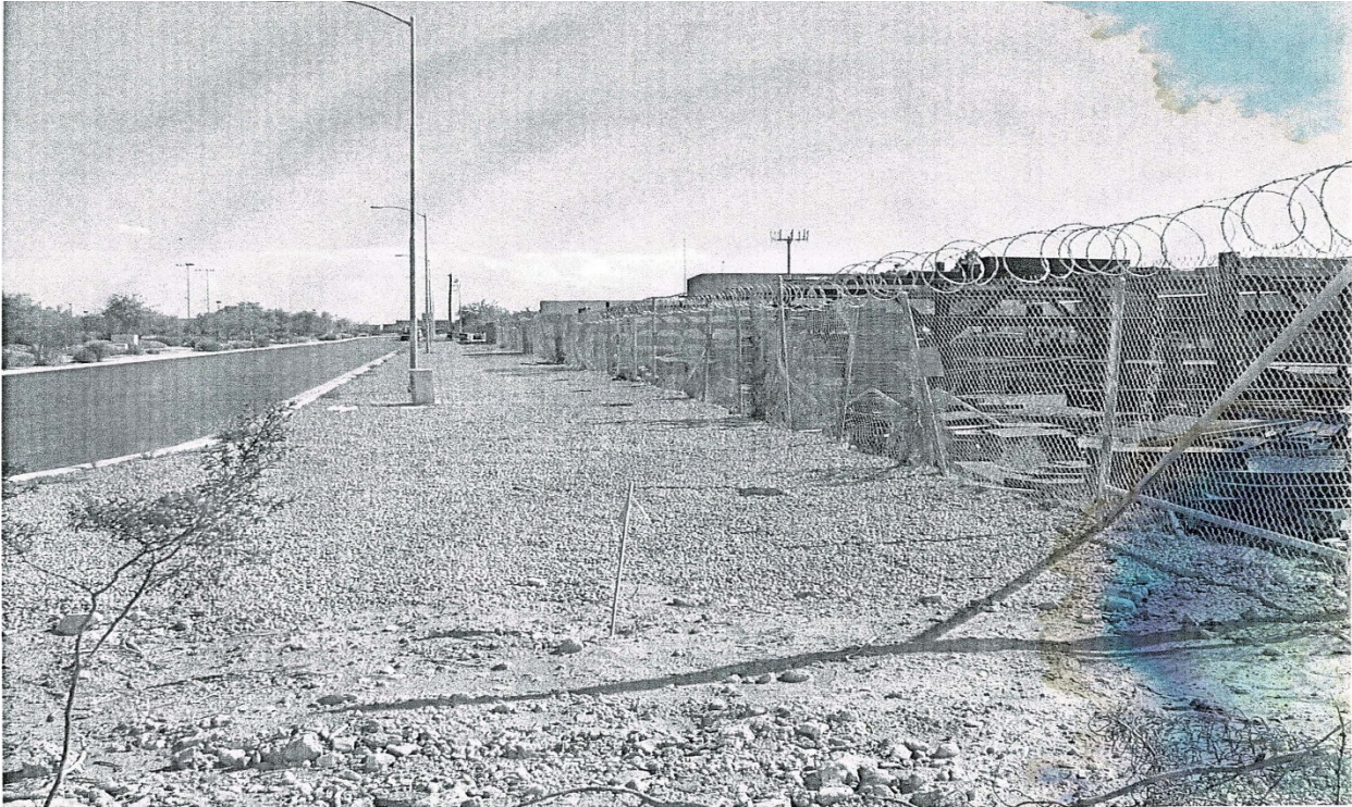
Figure 2 – West Side of Norwalk Before (North View)
