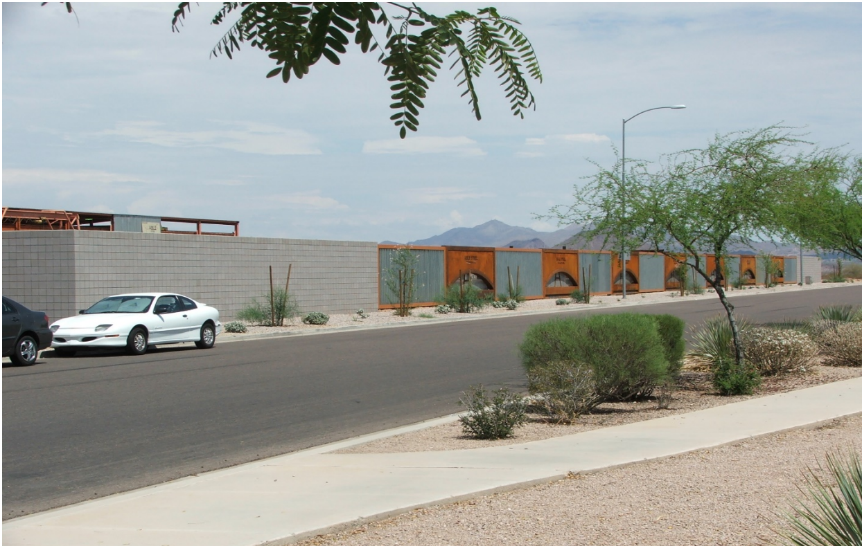
Figure 3 – West Side of Norwalk After (South View)
