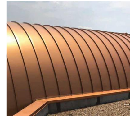
Copper Vauled Roof Standing Seam Metal Roof
