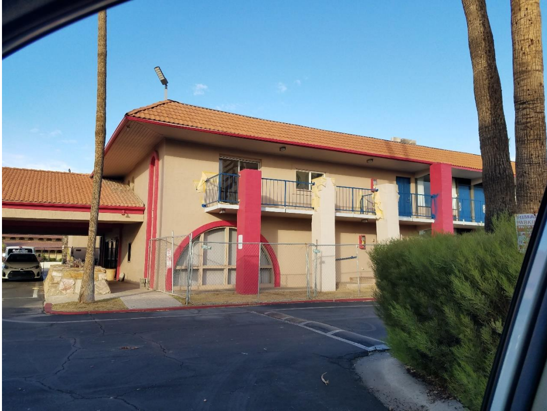
Southeast corner of Building 1
