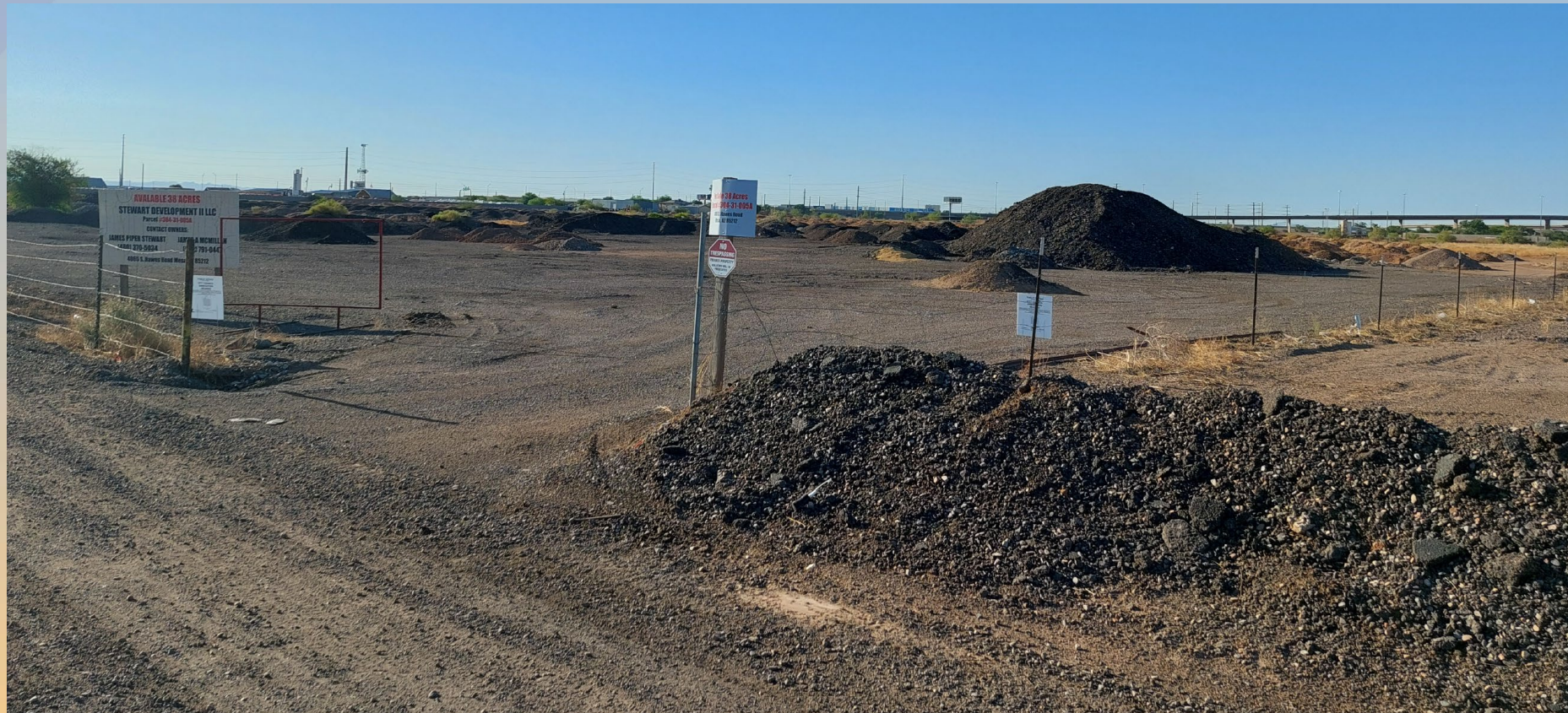
Looking southeast towards the project site from Mesquite Street
