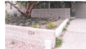
SANDBLASTED GREY CONCRETE
