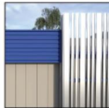
METAL PANELS PAINTED CENTURY BLUE METAL STUD SCREEN WALLS GALVANIZED FINISH
