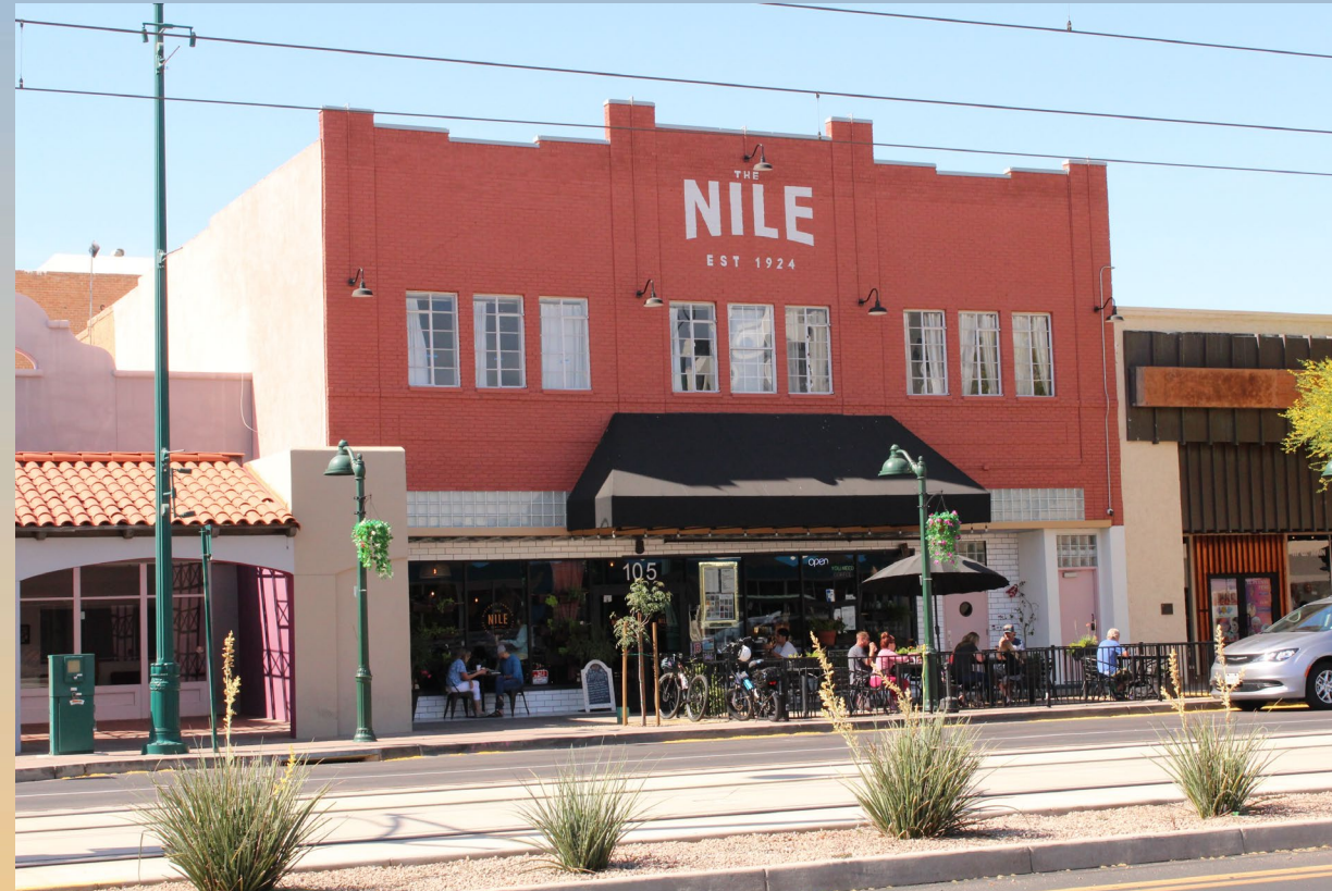
Looking south from Main Street
