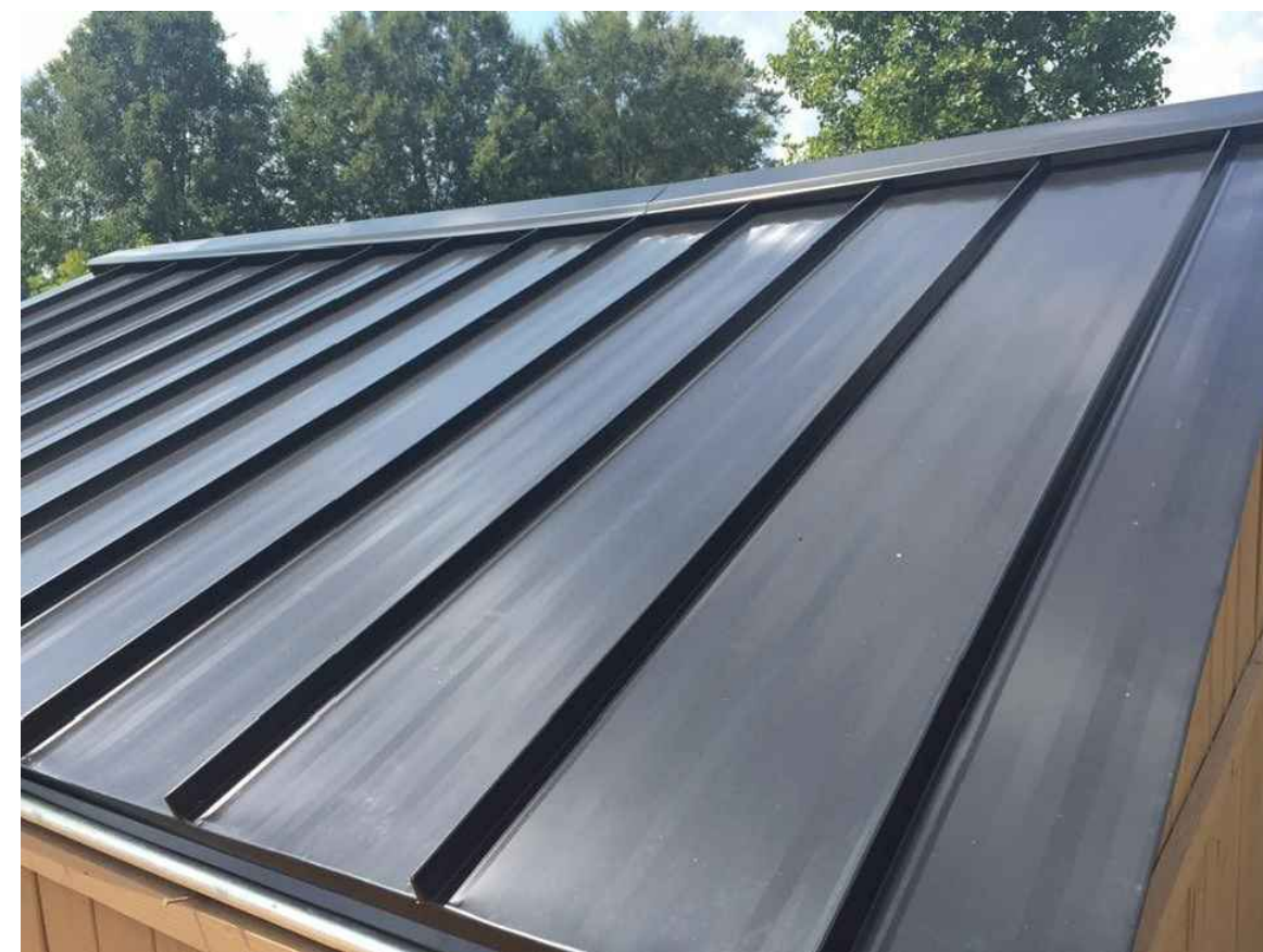
5 Standing Seam Roof SCALE: NTS
