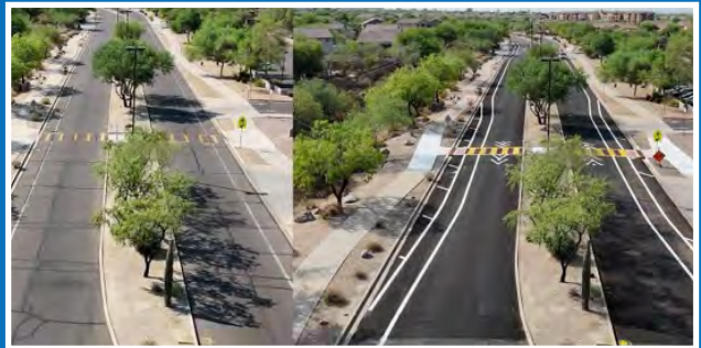
Las Sendas Elementary Raised Crosswalks
