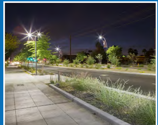
The Fiesta District Redevelopment Project incorporated safety improvements, such as landscape buffered sidewalks.
