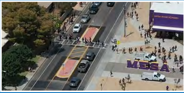
Mesa High School Pedestrian Refuge Island
