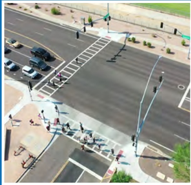
Highland Jr. High Traffic Signal (partially funded with photo safety funds)
